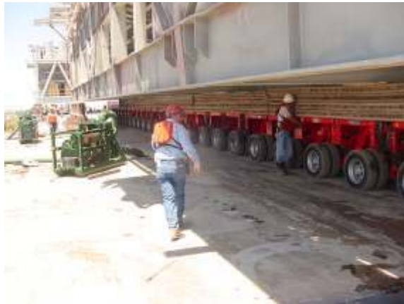
Pic. 59 PSP module transporter with drilling platform loaded
