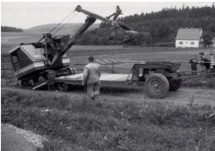
Pic. 5 First lowloader with rear-end loading, designed by Alois Goldhofer in 1952
